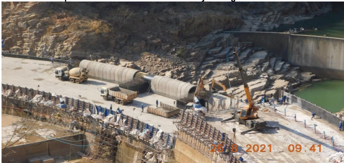
Preparation to Place Concrete on Gwayi Shangani dam wall
